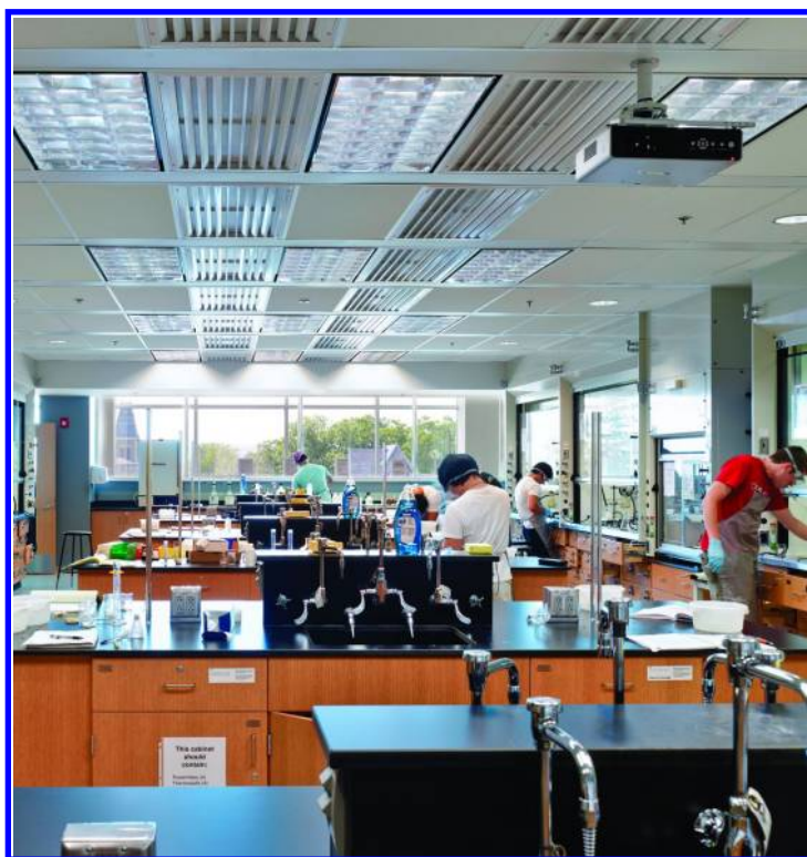
Figure 9. Two students can share 7-foot fume hoods at organic chemistry labs in Cornell University's Physical Sciences Building. (photo courtesy of Jeffrey Totaro). (see color insert)
