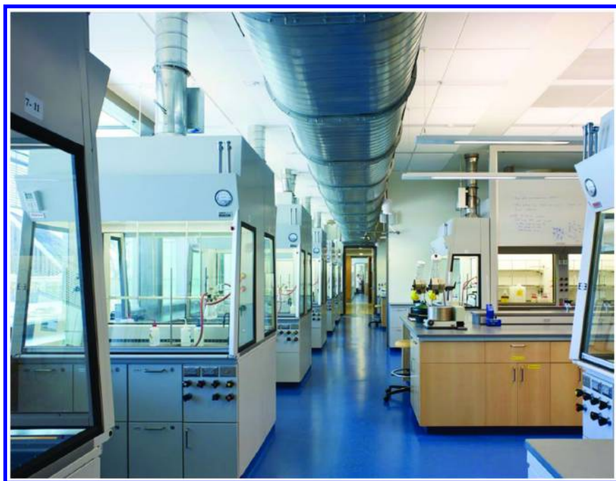
Figure 3. Princeton University, Frick Chemistry Laboratory: Introductory chemistry teaching laboratory with individual fume hoods per student and open passages between lab modules. Payette, Architect, in collaboration with Hopkins Architects, Design Architect Image Credit: © Warren Jagger Photography. (see color insert)
